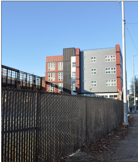
Rainier Ave. at the Mt. Baker Station
